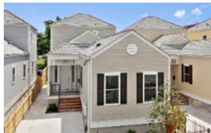
NORA; Saratoga Development Cost $1,546,363 2000SF Constructions of Energy Star and Green Communities.
