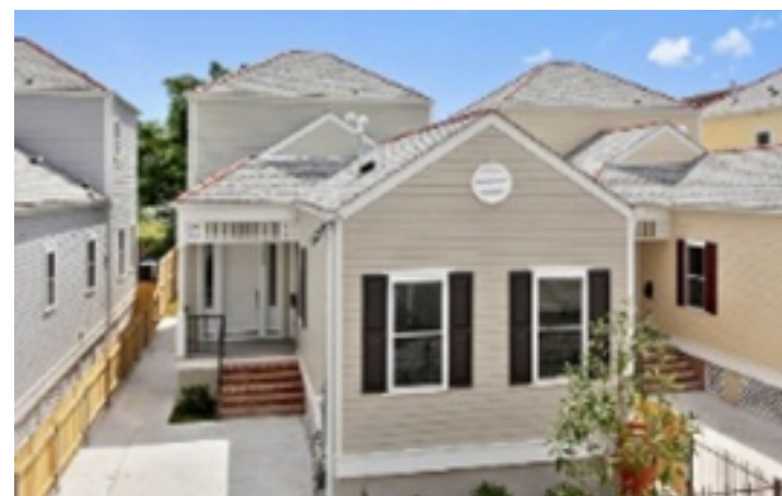
NORA; Saratoga Development 2000SF Constructions of Energy Star and Green Communities.
