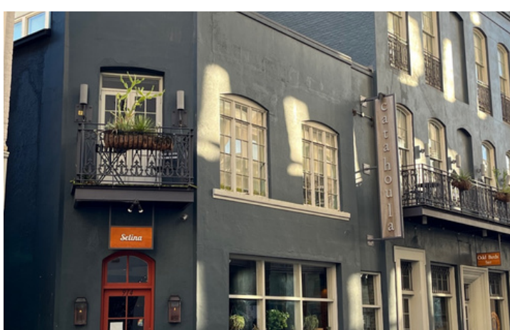
Catahoula Hotel Partial renovation of 15,000SF hotel.
